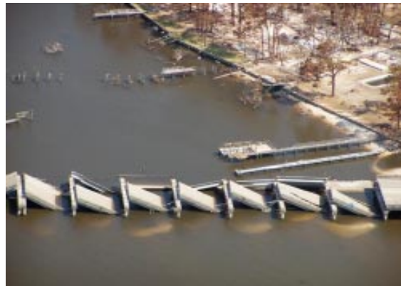
The superstructure units for the US 90 bridge at the east end of St. Louis Bay in Mississippi have been displaced to the north and many have dropped off the piers. The failure pattern is typical of what has been witnessed in past earthquakes.
