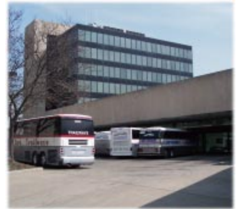
Bus terminal of Niagara Frontier Transportation Authority in Buffalo.
