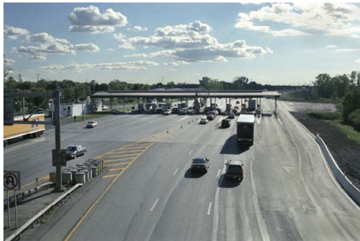
Lackawanna Toll Barrier – Milepost 430.5 NYS Thruway
