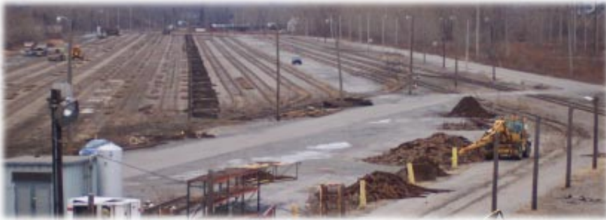
Photo at left shows CSX Railroad’s modification last fall of Seneca Yard in Lackawanna to serve as a “Feeder Port” to handle overseas container traffic shipped by rail from overwhelmed Port of New York and New Jersey. Layout of tracks was modified to accommodate cranes to unload and store containers for further transport by trucks. Work on modifications will continue in the spring. Regional economists see project as opportunity for warehousing or assembly plants associated with distribution of imported goods to Ontario, Midwest and other markets.
