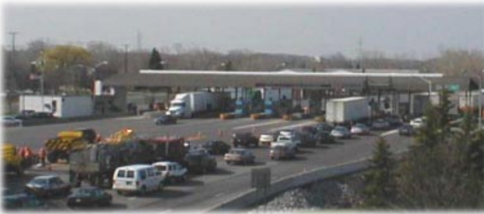
A traffic scene at the Lackawanna Toll Barrier.
