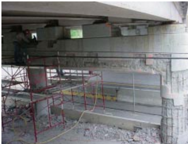
An example of bridge reconstruction on I-290.
