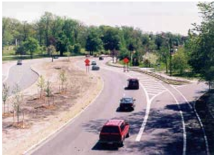
Delaware Avenue “S” curves designed by Olmsted.
