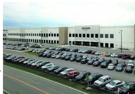
Amazon distribution facility near Cleveland was built on the site of the Randall Park Mall, which closed in 2009. Source: Retail-to-Warehouse Conversions Gain Momentum, NAIOP
