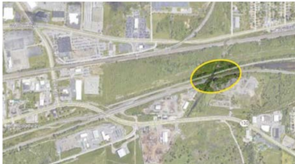
Aerial view of Structurally Deficient Bridge
