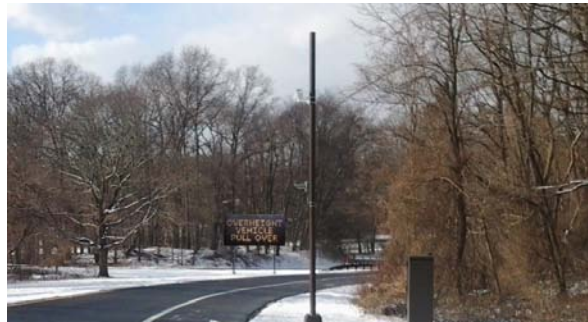
Example of low bridge clearance warning detection system in operation in Long Island. Source: NYSDOT.
