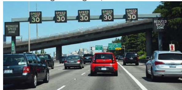
Example of variable speed limits and queue warnings. Source: NITTEC
