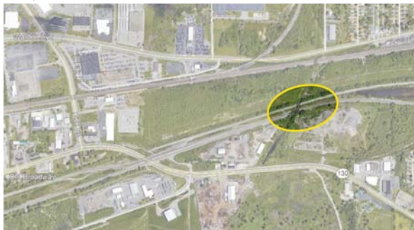
Aerial view of Structurally Deficient Bridge
