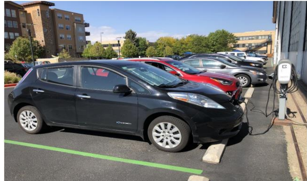
Community EV Charging (Source: Erik Nelsen / ICF) - Top
